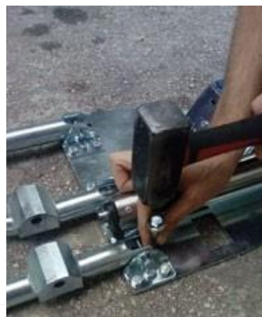
Figure 10 – Placer les ancrages
